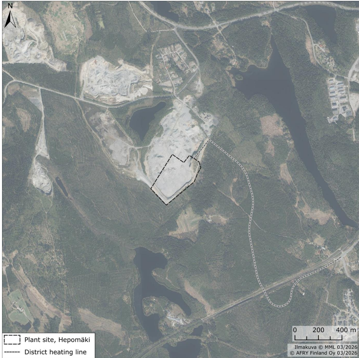
Figure 15-1. Aerial view of the Hepomäki (VE1) SME plant area and district heating transmission line area.
